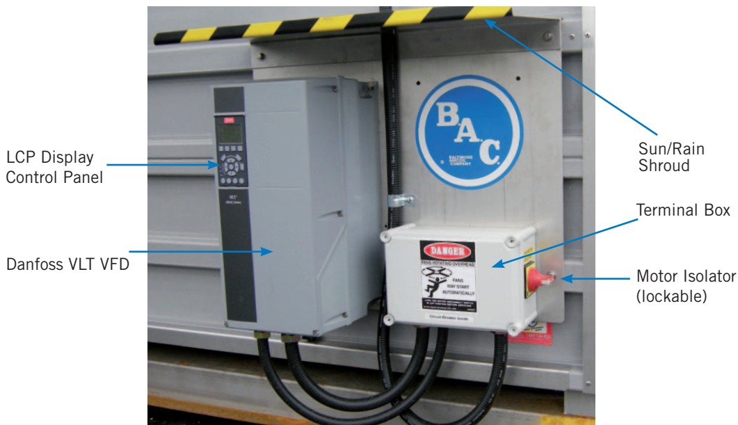
Figure 2. BAC Intelevap Controller Assembly
